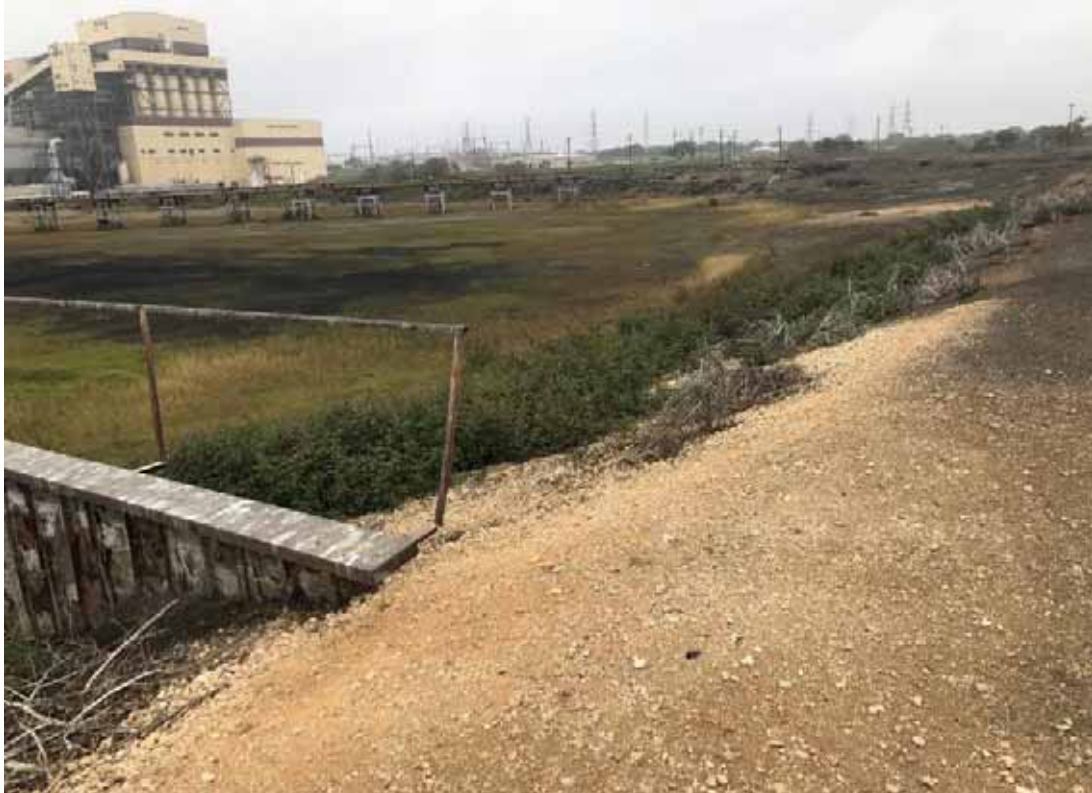
Photograph: 29 South Bottom Ash Pond – standing on southeast corner – facing northwest. Photo taken 12/14/2021.
