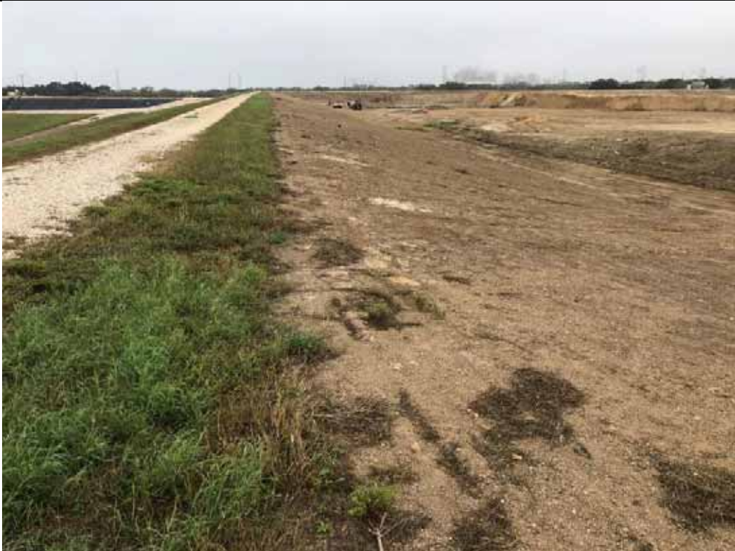
Photograph: 5 Fly Ash Landfill – standing on northeast corner – facing south. Photo taken 12/14/2021.
