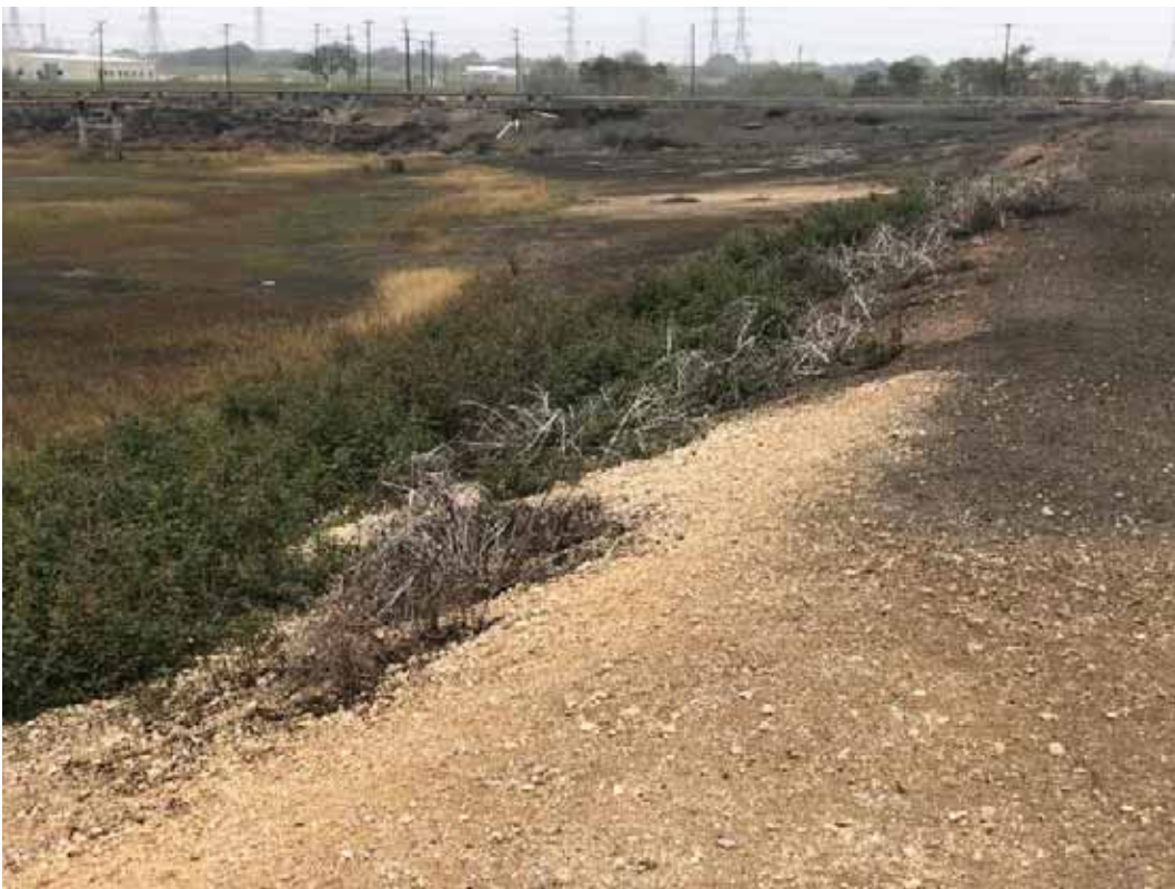
Photograph: 28 South Bottom Ash Pond – standing on southeast corner – facing north. Photo taken 12/14/2021.
