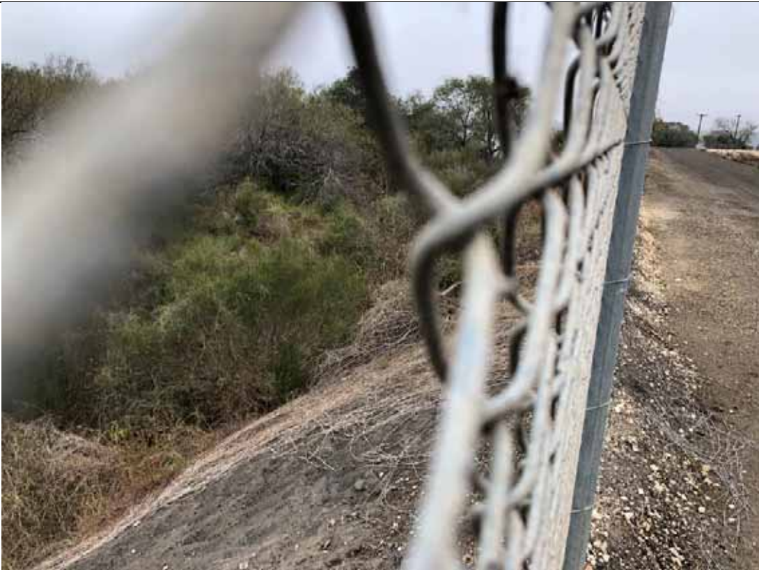
Photograph: 19 North Bottom Ash Pond – standing on northwest corner – facing east. Photo taken 12/14/2021.
