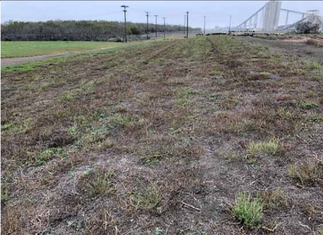
Photograph: 27 South Bottom Ash Pond – standing on northeast corner – facing south. Photo taken 12/14/2021.
