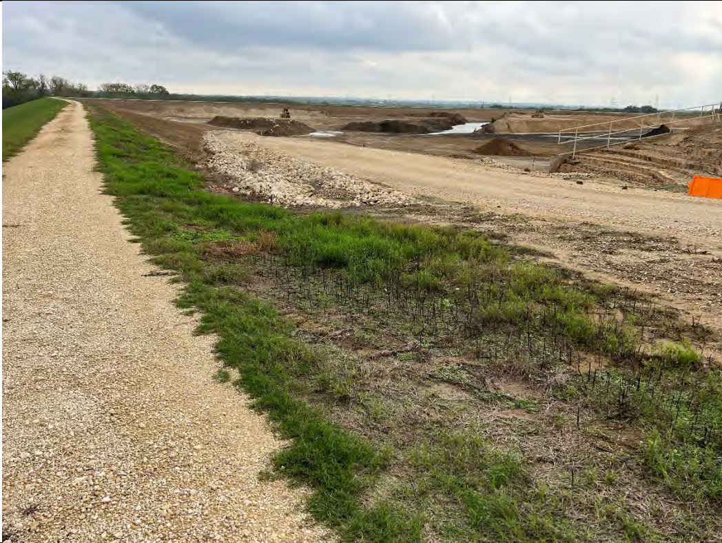
Photograph: 1 Fly Ash Landfill – standing on northwest corner – facing east. Photo taken 12/13/2022.
