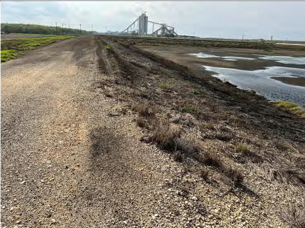
Photograph: 22 | North Bottom Ash Pond – standing on northeast corner – facing south. Photo taken 12/13/2022.
