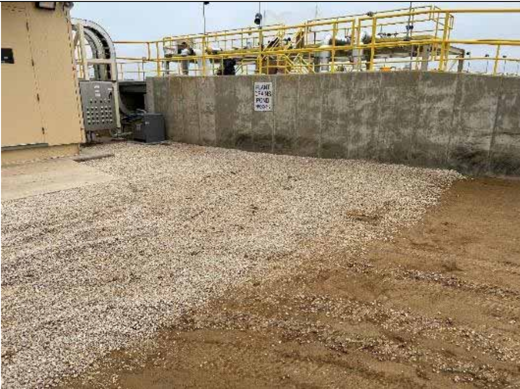
Photograph: 52 Plant Drains Pond – standing on the north side of ponds – facing south. Photo taken 11/16/2023.
