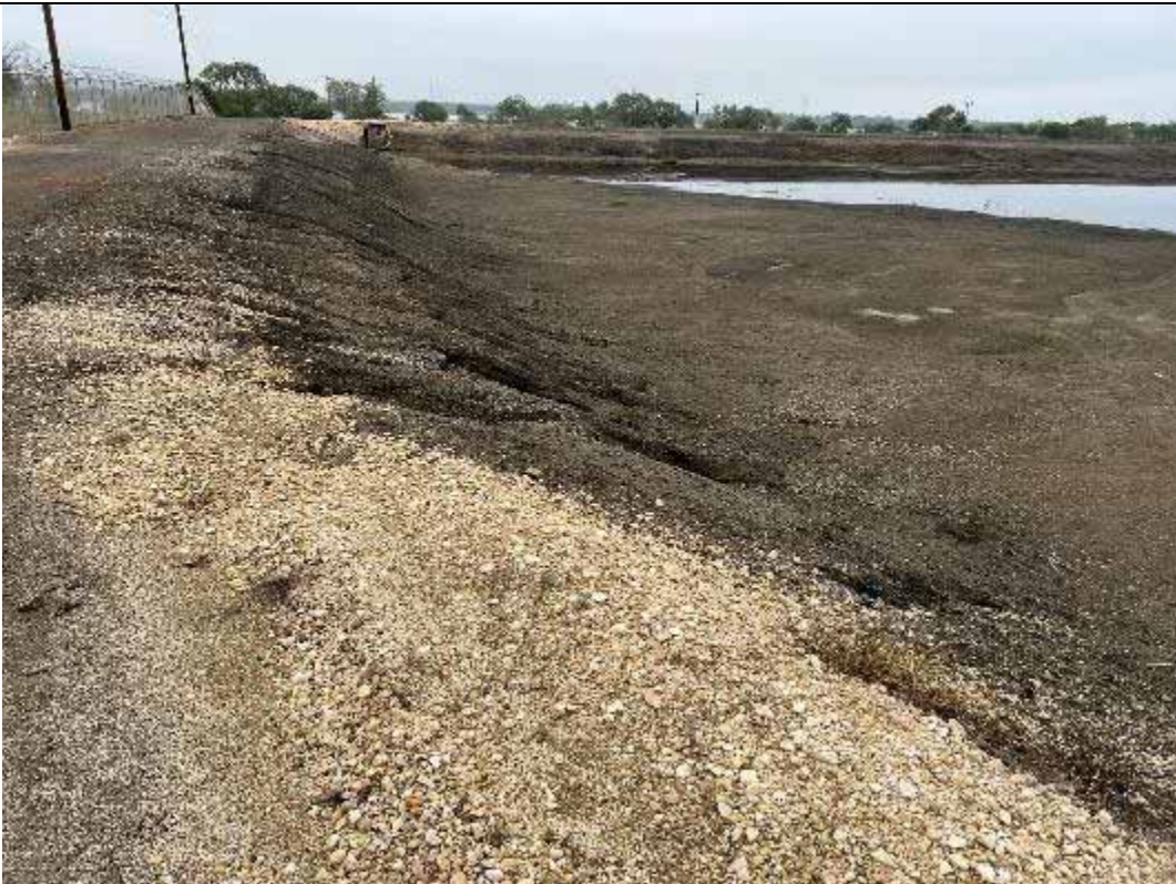
Photograph: 20 North Bottom Ash Pond – standing on northwest corner – facing east. Minor erosion noted on the north interior slope. Photo taken 11/16/2023.
