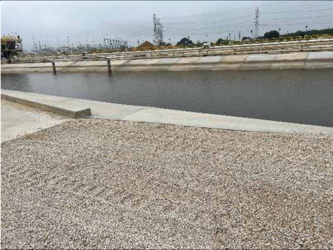
Photograph: 53 East Plant Drains Pond – standing on the east side – facing west. Photo taken 11/16/2023.
