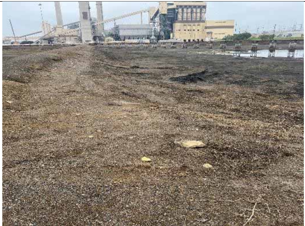
Photograph: 26 North Bottom Ash Pond – standing on southeast corner – facing west. Photo taken 11/16/2023.
