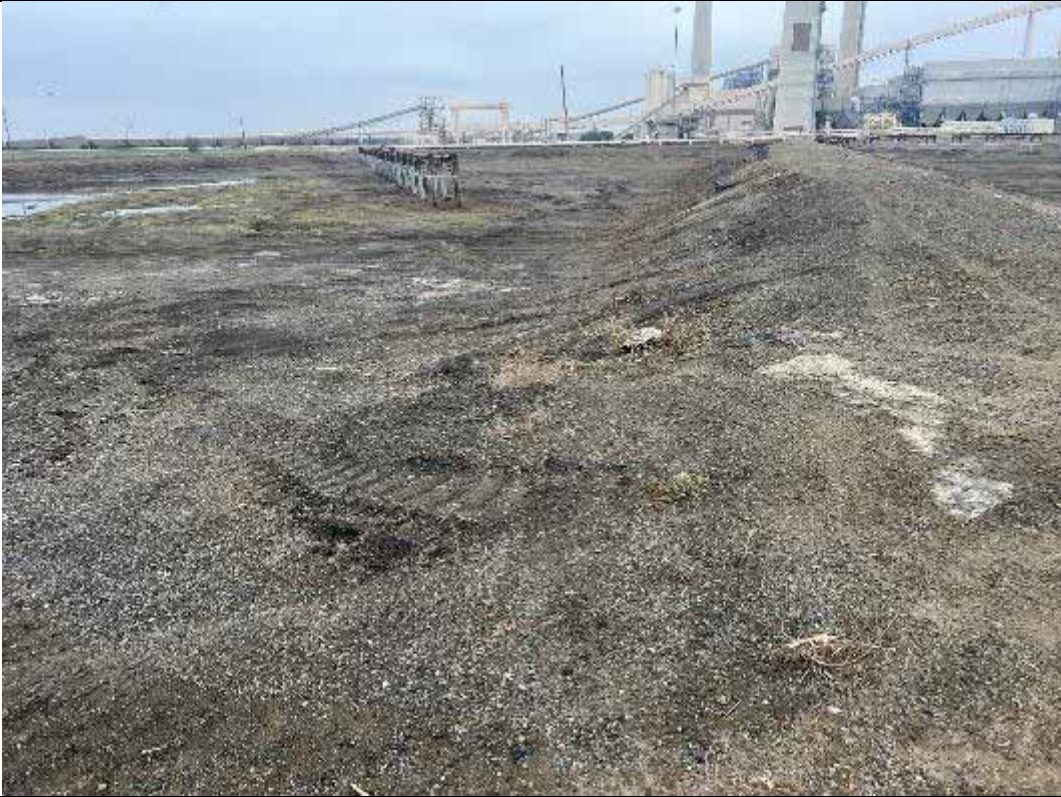
Photograph: 27 South Bottom Ash Pond – standing on northeast corner – facing west. Photo taken 11/16/2023.
