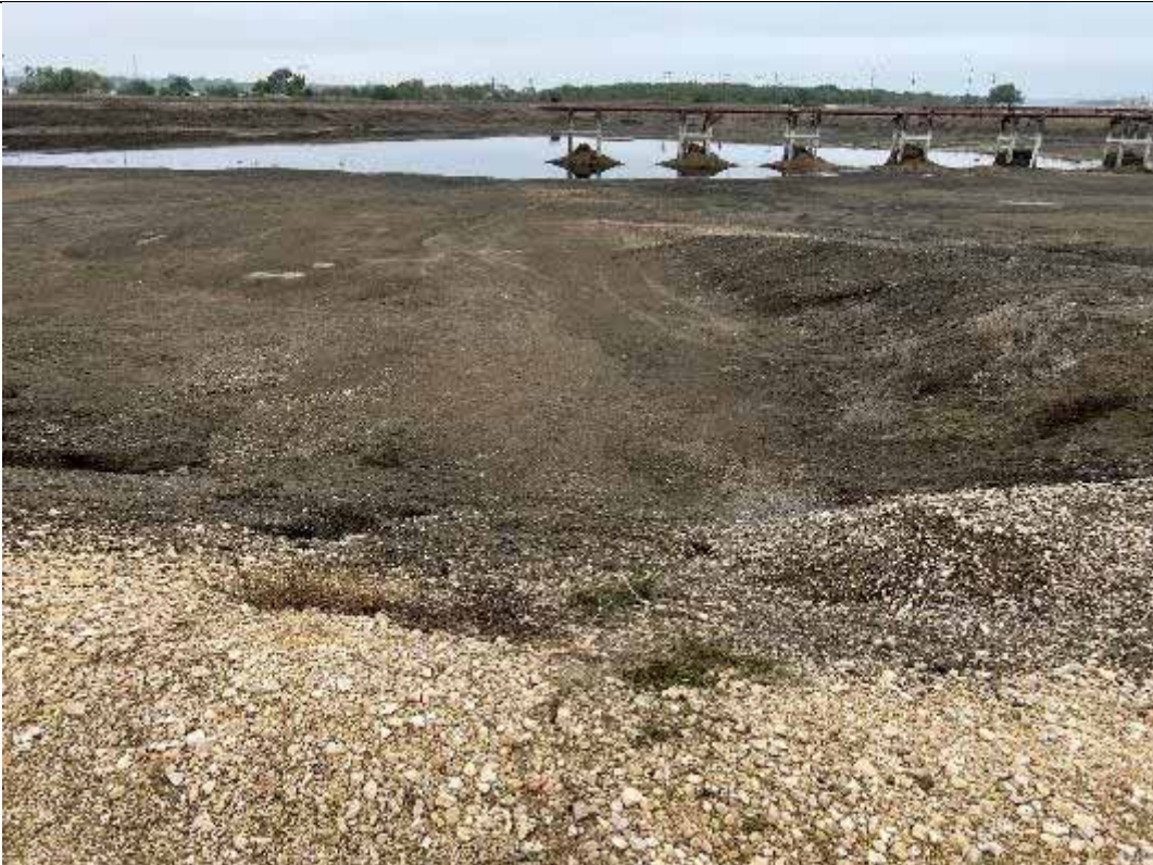
Photograph: 23 | North Bottom Ash Pond – standing on northwest corner – facing southeast. Photo taken 11/16/2023.
