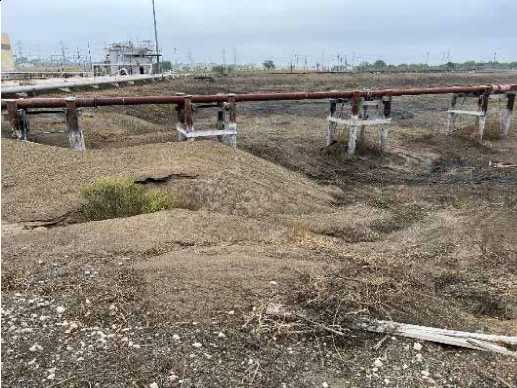
Photograph: 29 South Bottom Ash Pond – standing on southwest corner – facing north. Photo taken 11/16/2023.
