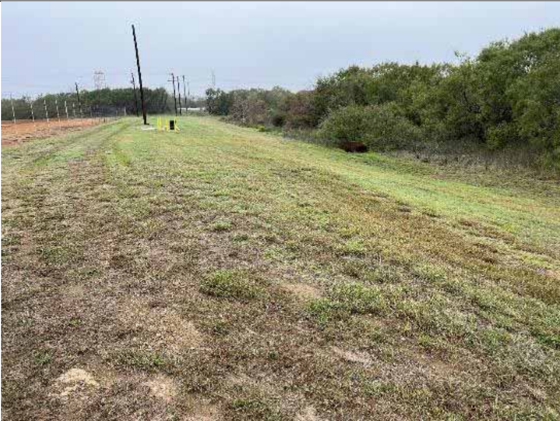
Photograph: 11 Evaporation Pond – standing on the northeast corner – facing west. Photo taken 11/16/2023.
