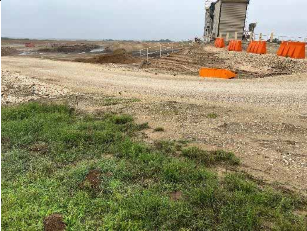
Photograph: 3 Fly Ash Landfill – standing on northwest corner – facing south. Photo taken 11/16/2023.
