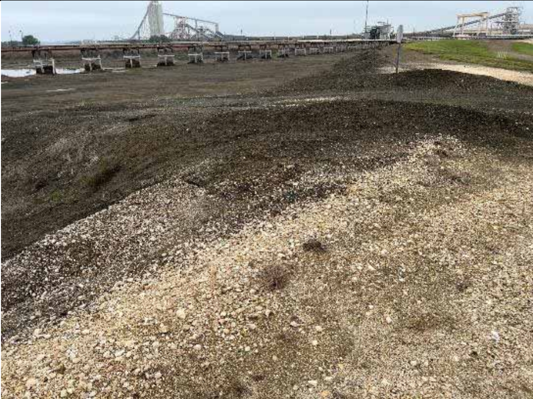
Photograph: 21 North Bottom Ash Pond – standing on northwest corner – facing south. Photo taken 11/16/2023.
