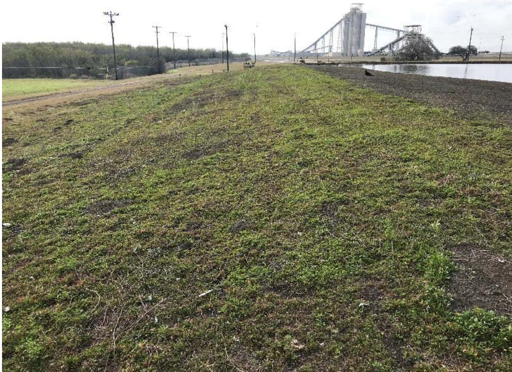
Photograph: 23 South Bottom Ash Pond – standing on eastern berm – facing south. Photo taken 12/18/18.
