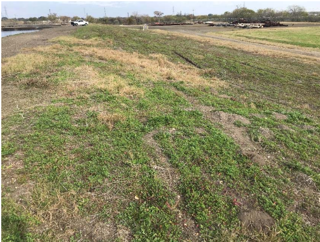
Photograph: 24 South Bottom Ash Pond – standing on eastern berm – facing north. Minor rutting due to vehicle traffic noted on eastern berm exterior side slope. Photo taken 12/18/18.
