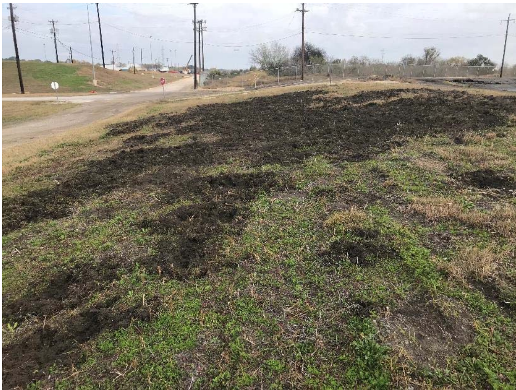
Photograph: 22 | North Bottom Ash Pond – standing on western berm – facing north. Surficial vegetation damage due to hog activity. Photo taken 12/18/18.
