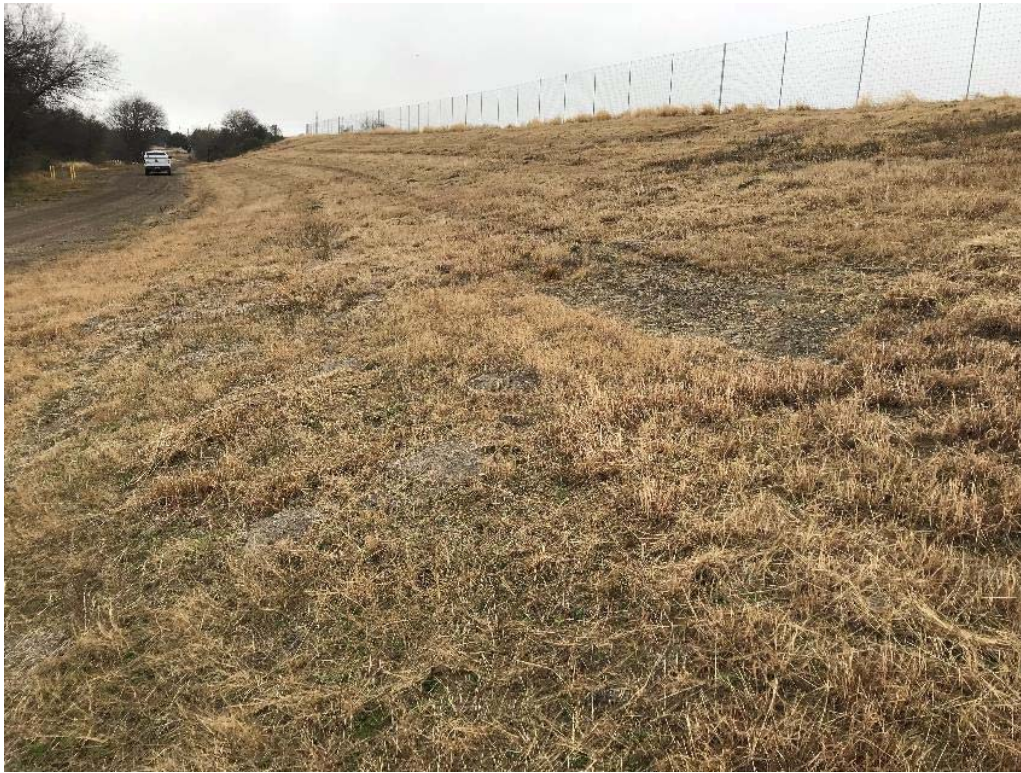
Photograph: 15 Evaporation Pond – standing outside the northeast corner – facing south. Photo taken 12/18/18.
