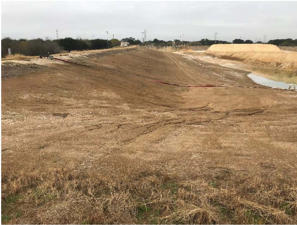
Photograph: 3 Fly Ash Landfill – standing on eastern berm – facing west. Radial stacker located in southwest corner of landfill. Photo taken 12/18/18.
