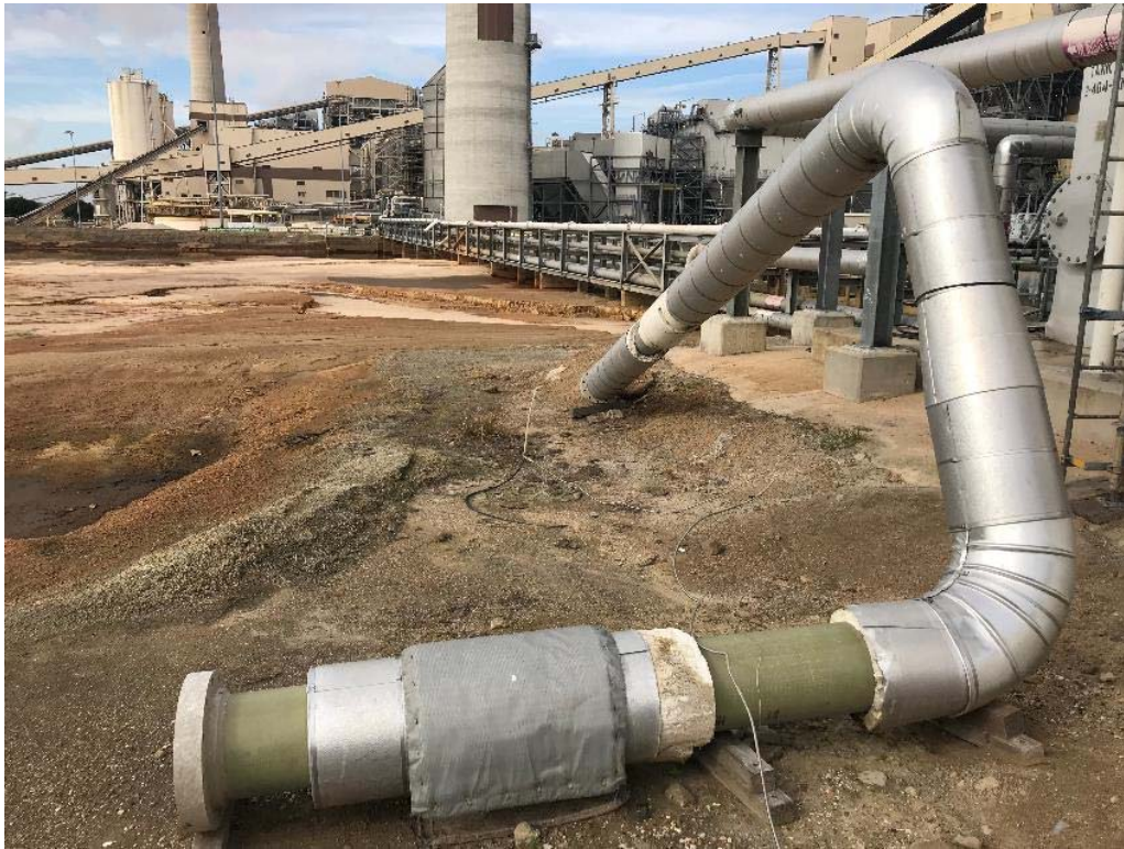
Photograph: 39 South SRH Pond – standing on the eastern berm – facing west. Substantially full of solids and not in use. Photo taken 12/18/18.
