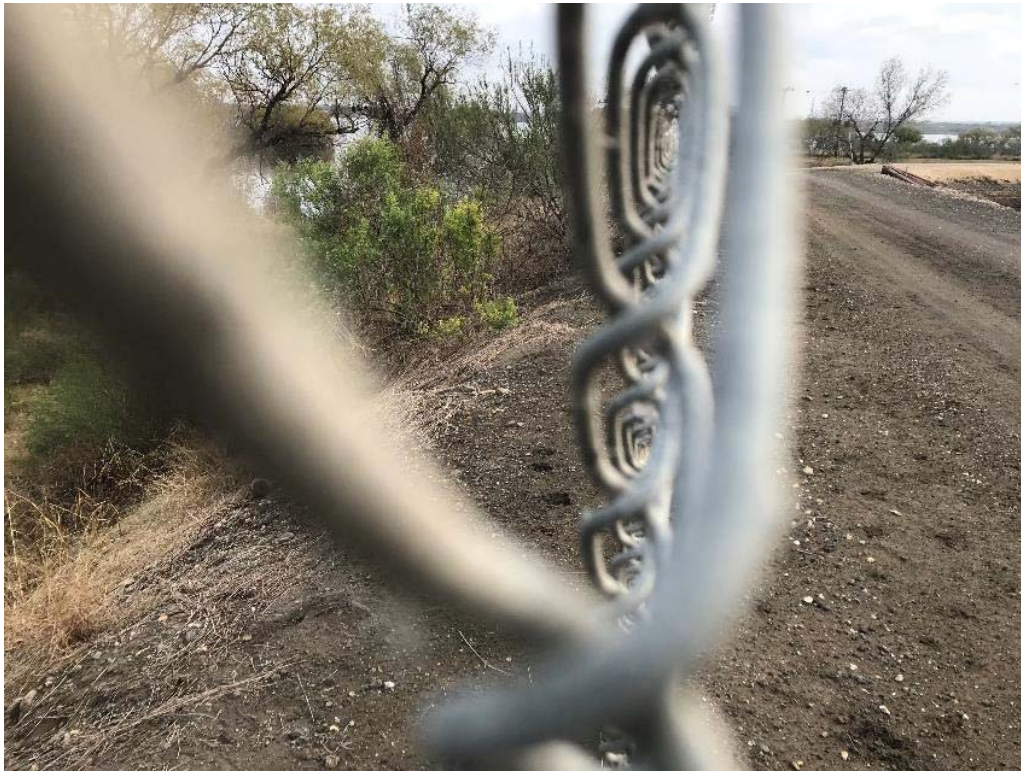
Photograph: 21 | North Bottom Ash Pond – standing on northern berm – facing east. Woody plant growth noted on northern berm exterior side slope. Photo taken 12/18/18.
