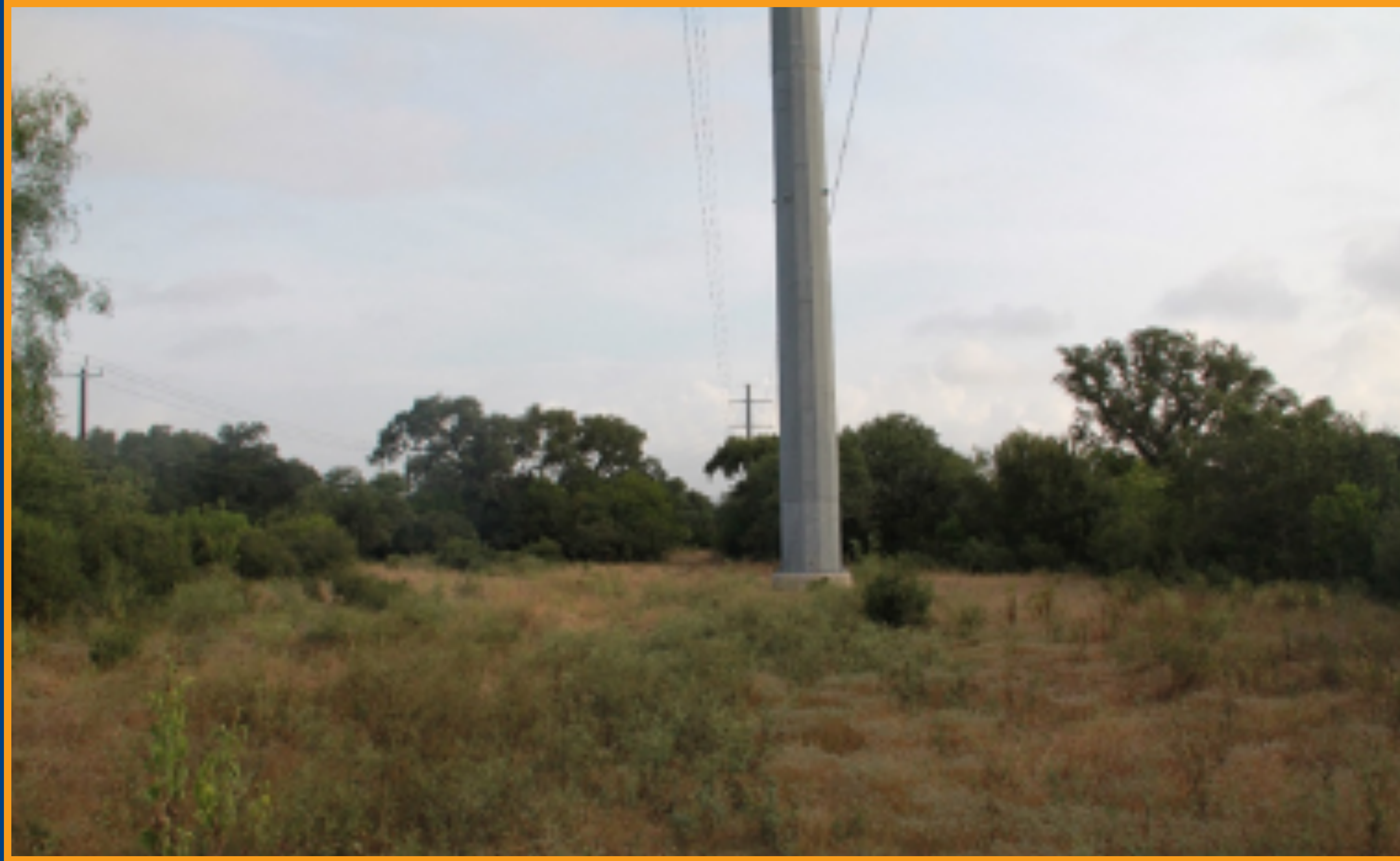
100 feet clearing around transmission structure
