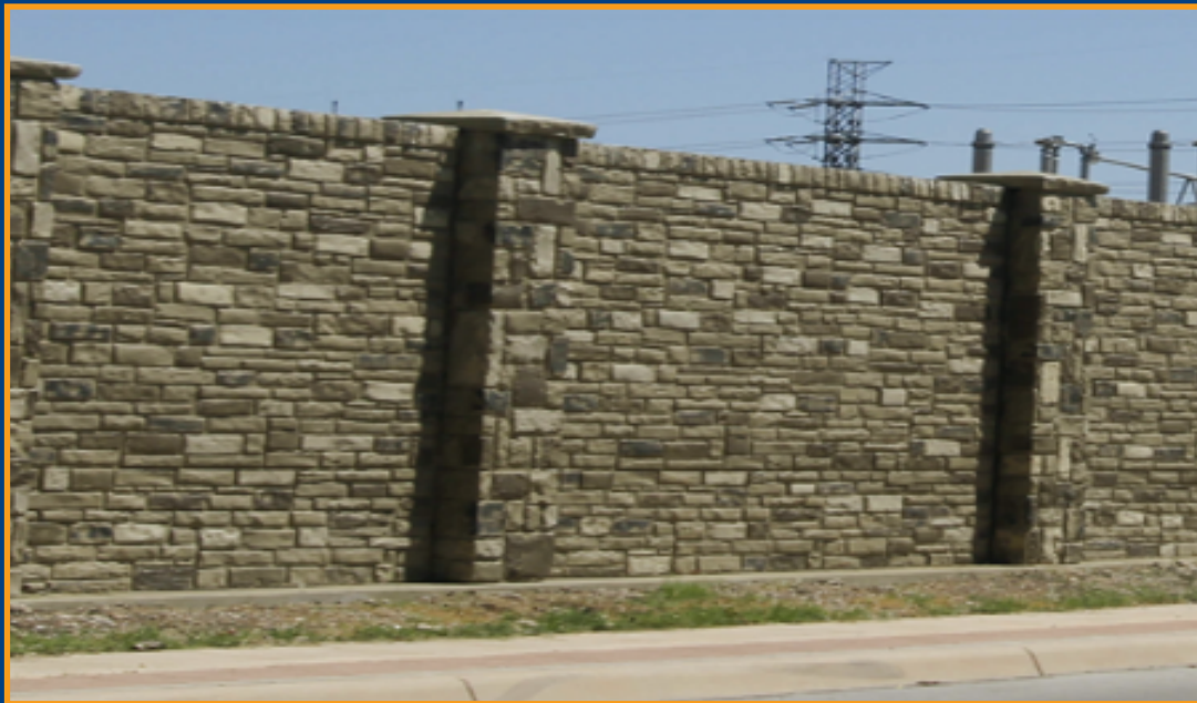
Ball Park Substation – Decorative concrete wall
