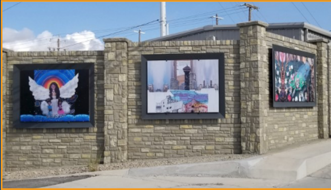
Dresden Substation – Decorative concrete wall (Art work provided by City of San Antonio)
