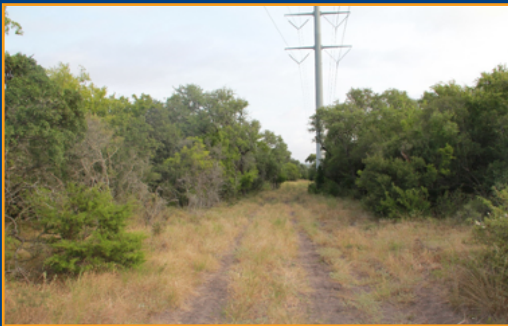
16-30ft clearing along route
