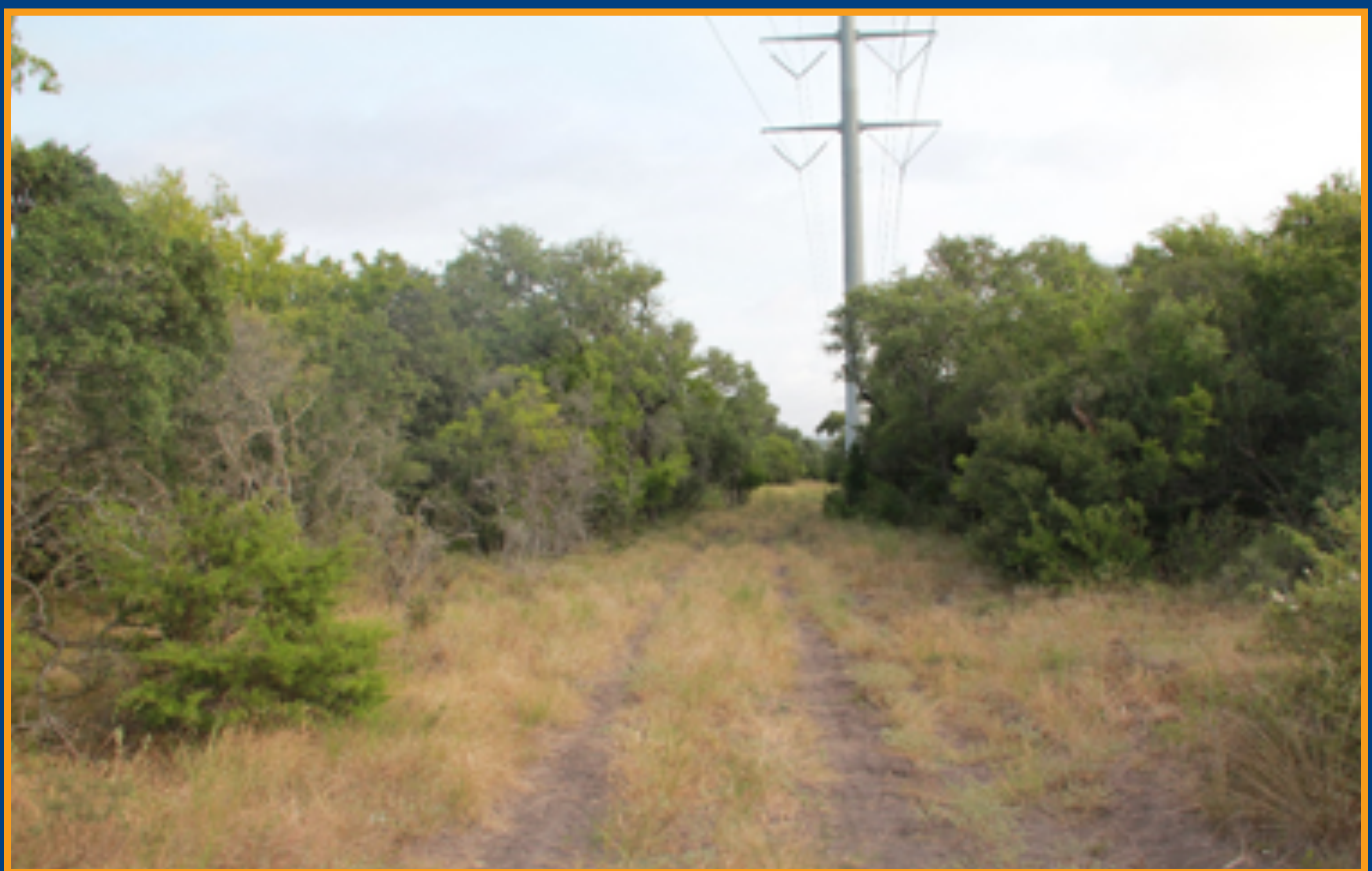
Clearing along route
