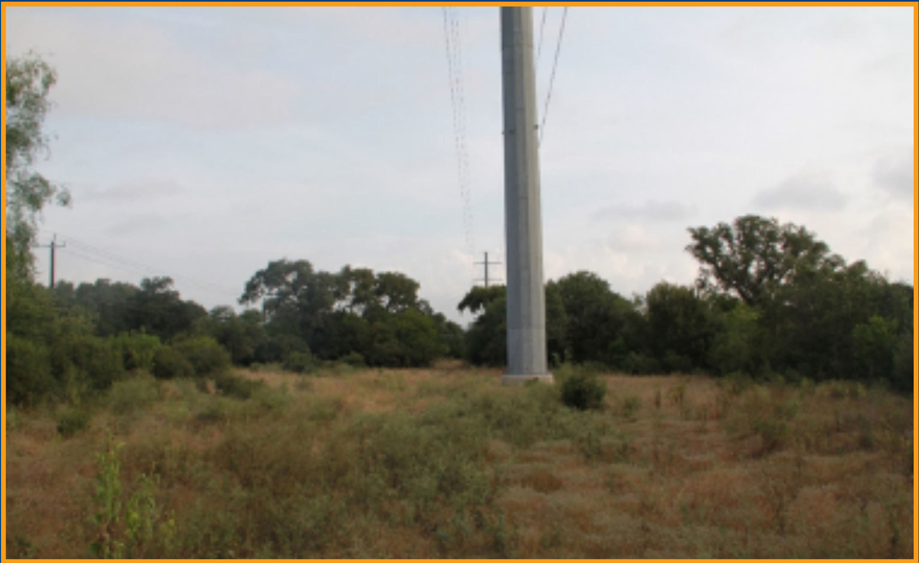
Clearing around transmission poles
