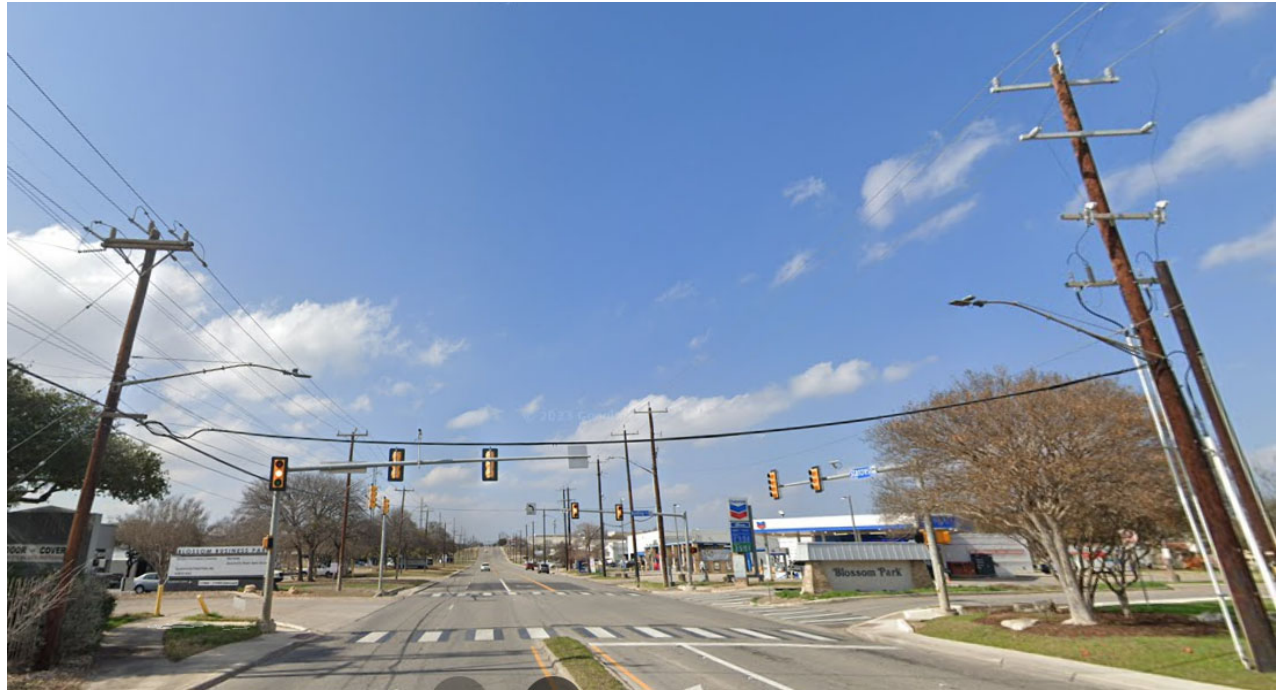
Communications don't follow existing power
