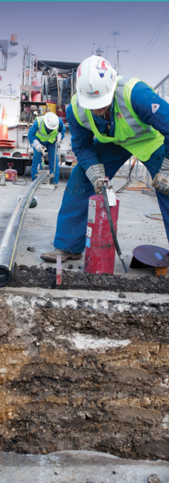
Gas Solutions team members work on underground infrastructure.
