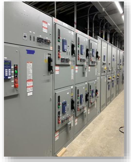
5kV Switchgear Upgrade
