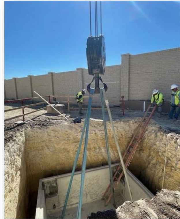
Our Contractor Setting a Manhole Outside a Substation
